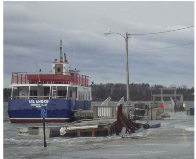
Inundation of Chebeague Island's Stone Pier
