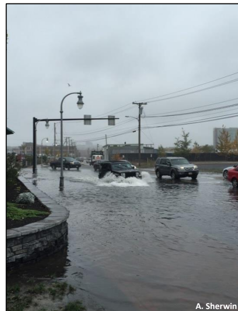
Nuisance flooding, like that seen here on Somerset Street in Portland during a high tide event, is predicted to become more frequent as precipitation increases and sea level rises.
