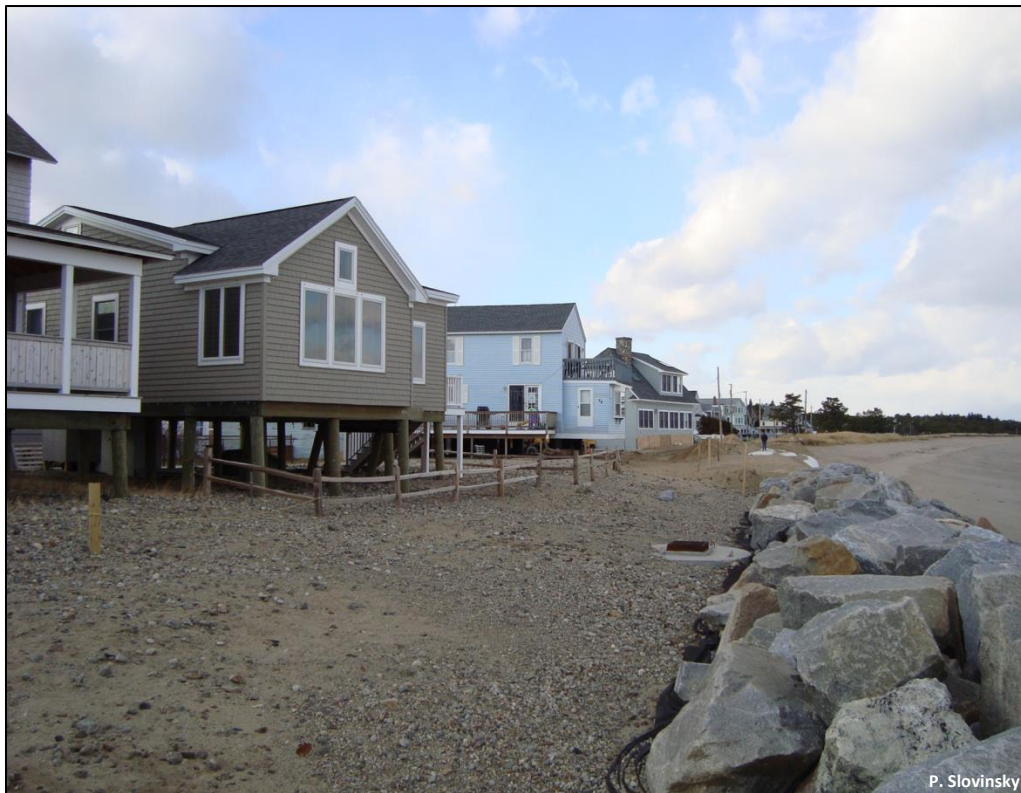
Elevating structures on pile foundations, seen here in the Camp Ellis neighborhood of Saco, protects structures against flooding, erosion, and scour.
