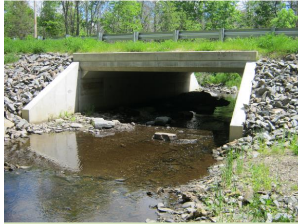
Restoring habitat connectivity at road crossings is an important conservation action for many SGCN and often involves coordination among state and local transportation agencies, biologists, landowners, and other partners. © John Perry
