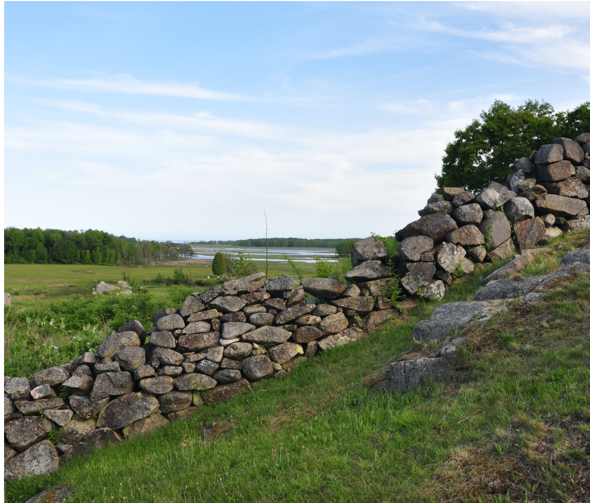
Stone Wall near Mills Road north of the Batson River
