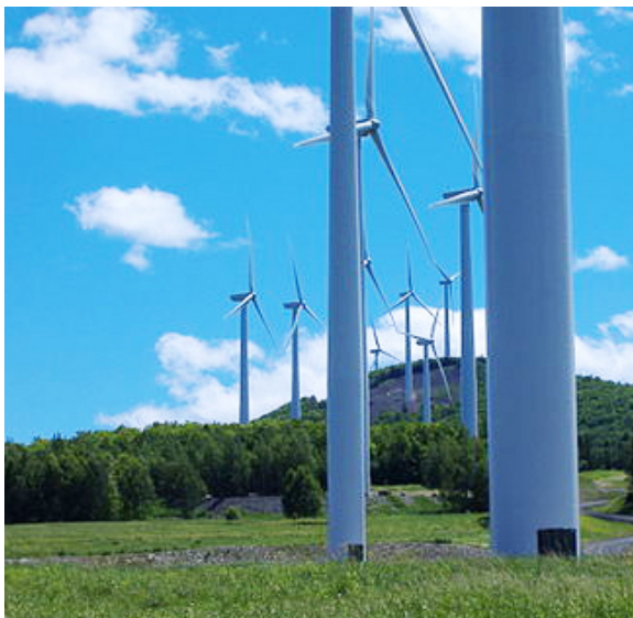
Several of the twenty-eight 1.5 MW wind turbines at the Mars Hill Wind Farm in the Saint John valley (Photo: Michael Surran)
