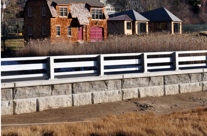
Village Seawall. Photo by Tom Morgan.
