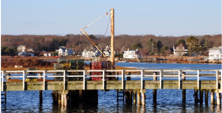
The Cape Porpoise Pier. Photo by Tom Morgan
