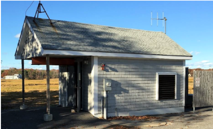
Pump Station #12, King’s Highway. Photo: Wright-Pierce.
