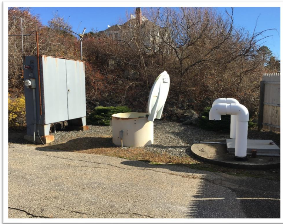
FIGURE 6 – OCEAN AVENUE PUMP STATION
