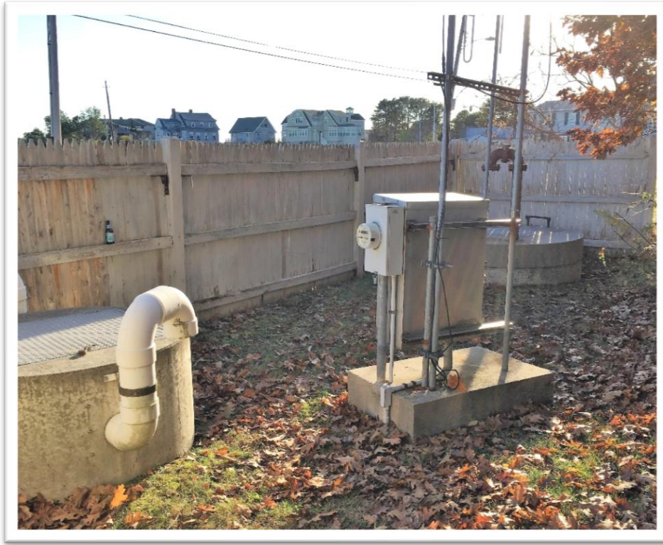
FIGURE 13 – KING’S LANE PUMP STATION
