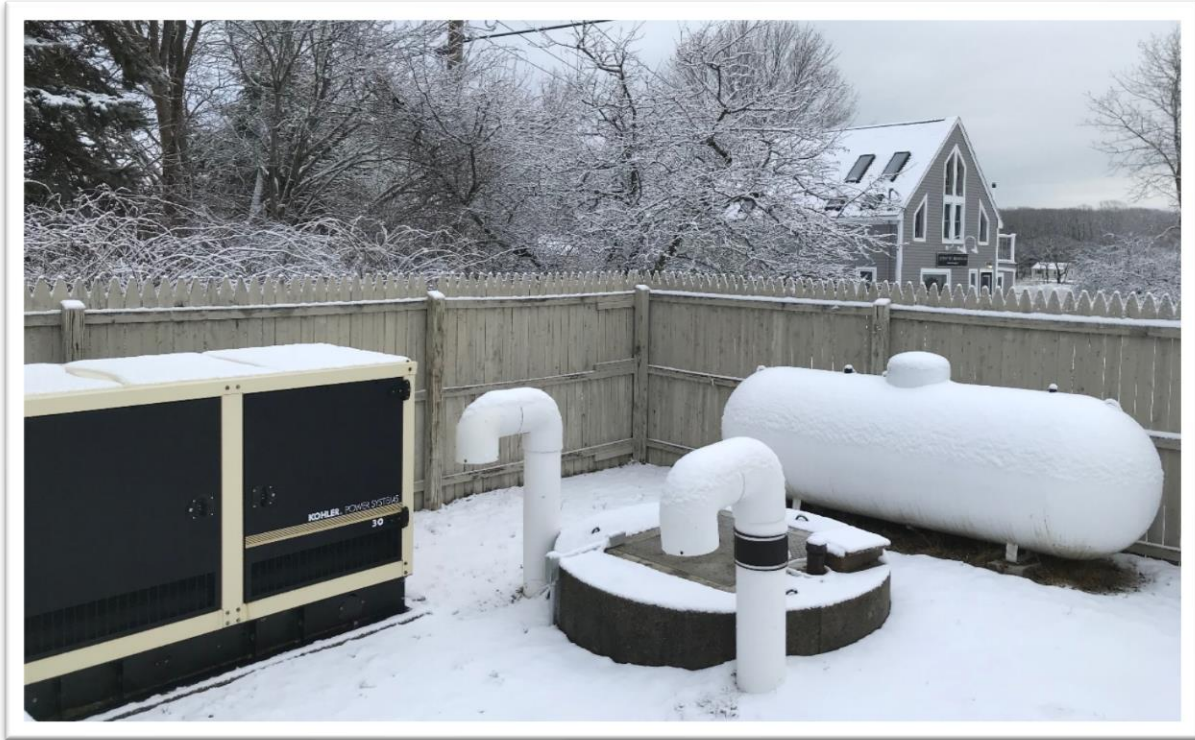
FIGURE 10 – CAPE SQUARE (PORPOISE) PUMP STATION
