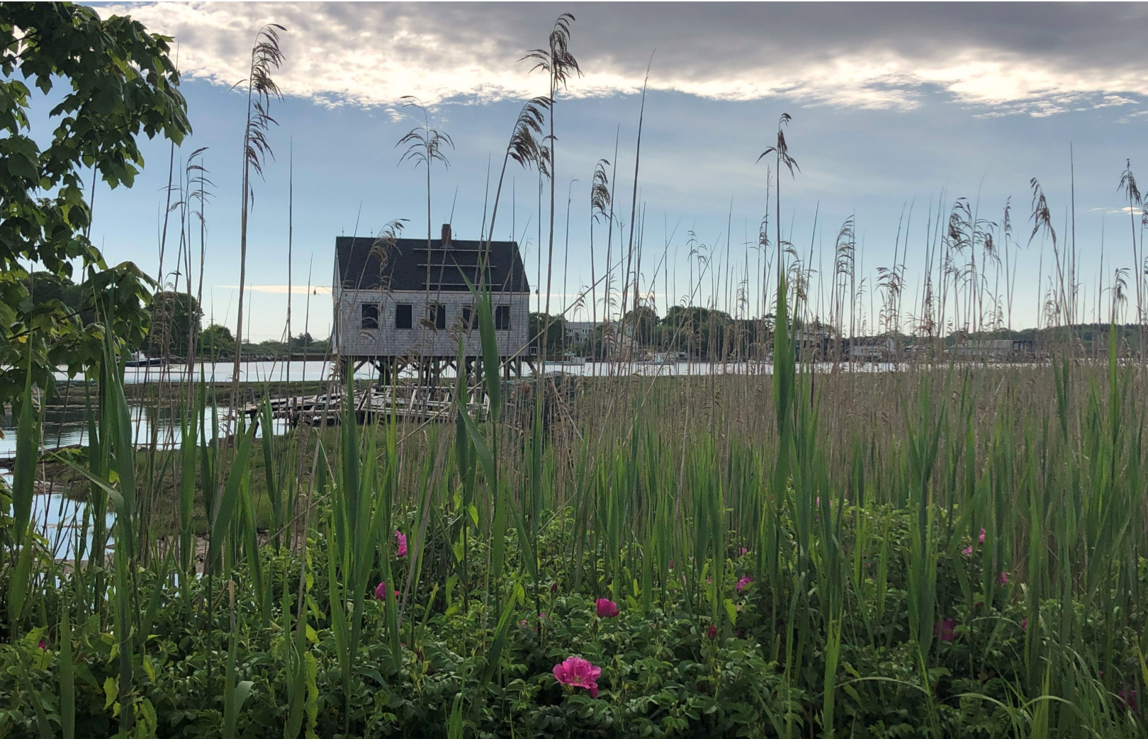
Elevated structure (L. Durfee)
