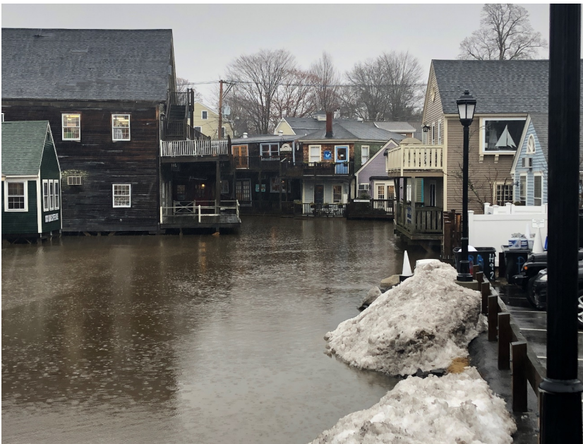
High water levels in Dock Square on Jan 20, 2021 (L. Durfee)
