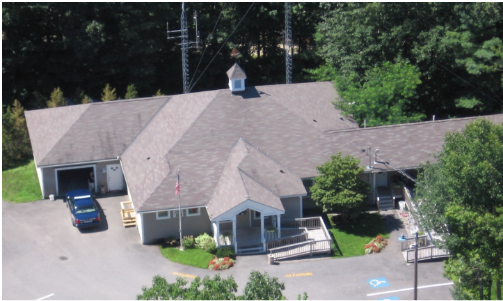
Kennebunkport Police Station. Photo courtesy of the Police Department.
