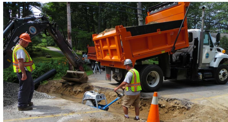
Culvert replacement on Turbats Creek Road. Photo courtesy of the Public Works Department
