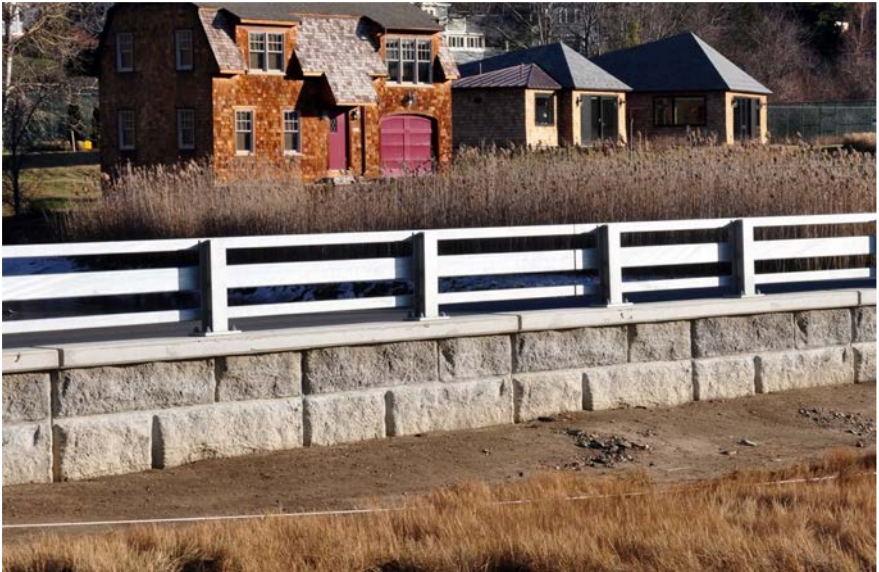
New seawall along Ocean Avenue 2021.
