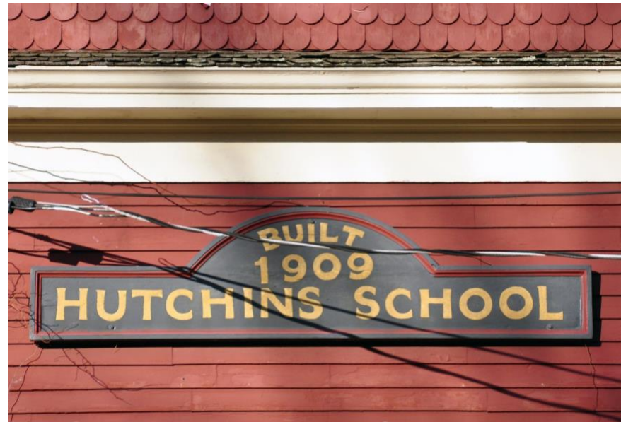
Educational standards have evolved since the former Hutchins School was erected in 1909. Photo: Tom Morgan
