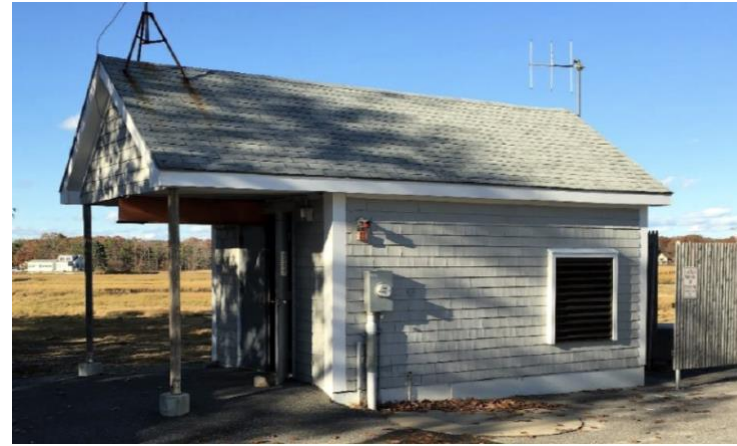
Pump Station #12, King's Highway. Photo: Wright-Pierce.
