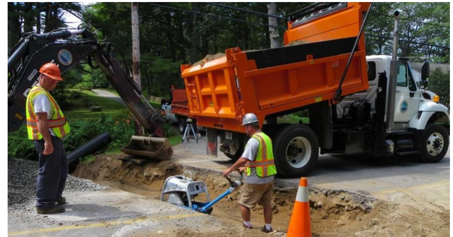
Culvert replacement on Turbats Creek Road. Photo courtesy of the Public Works Department.
