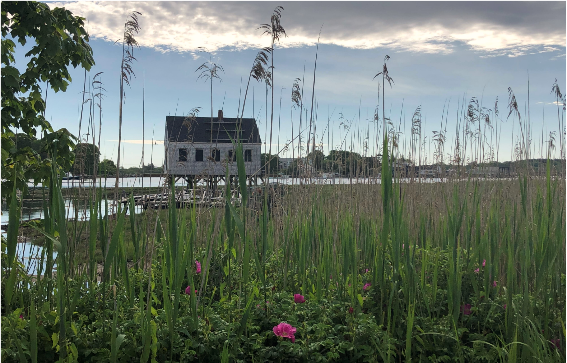
Elevated structure (E. Durfee)
