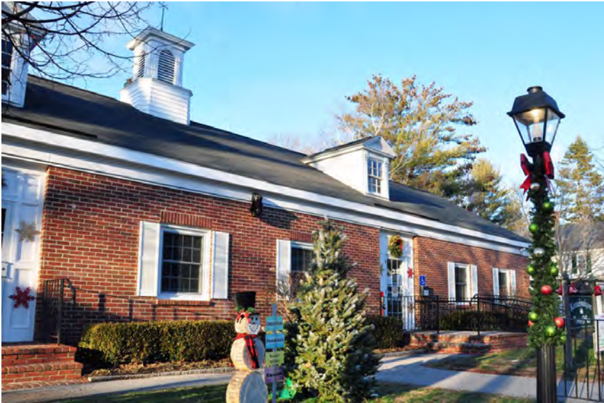
Town Offices at 6 Elm Street. Photo: Tom Morgan
