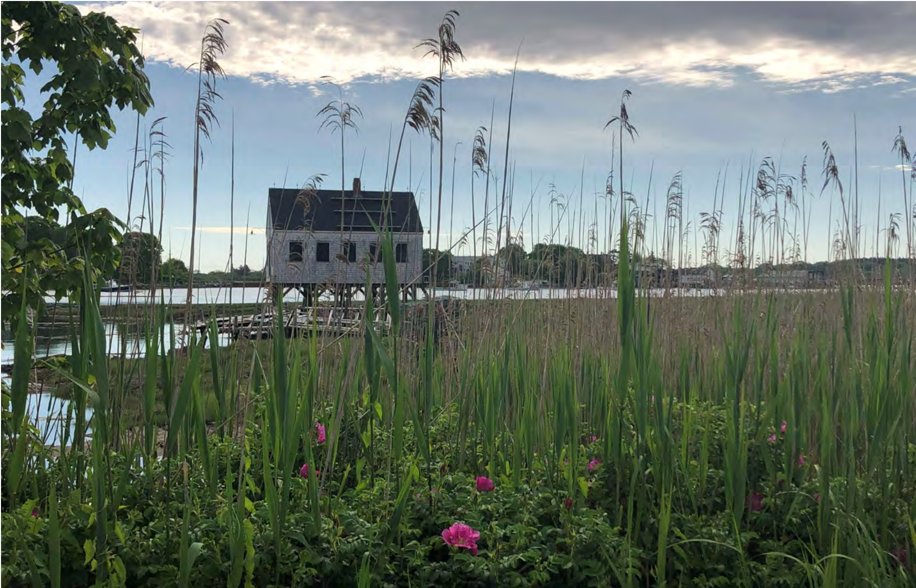
Elevated structure (E. Durfee)
