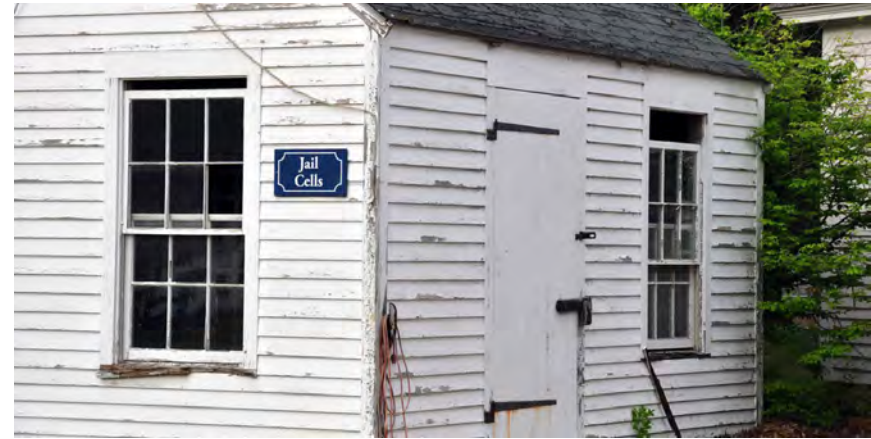
The old Lock-Up has been out of service for quite some time. Photo: Tom Morgan.
